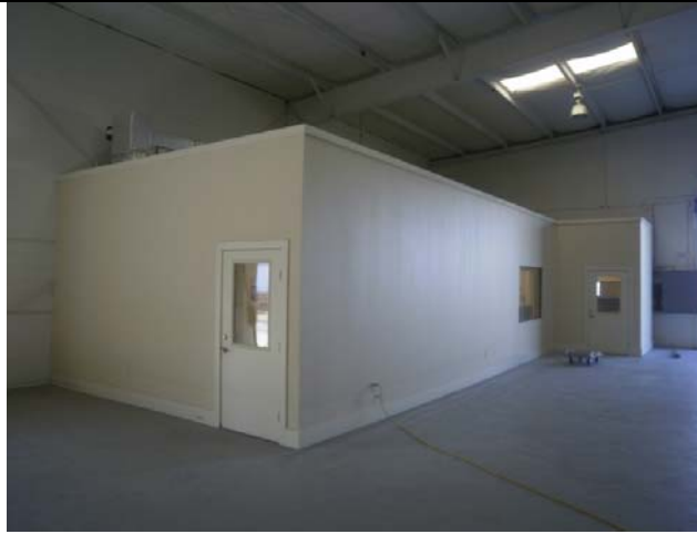
In warehouse added breakroom & bathrooms
