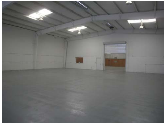
wall sheathing, painted walls & floor coating
